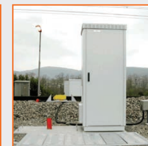
Axle counter, zone controller, wheel T°, track maintenance, interlocking.
