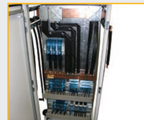
nVent integrated solution containing nVent HOFFMAN enclosure for wayside radio/fiber-optic management and nVent ERIFLEX low voltage power distribution products.
