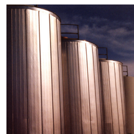
Tank Insulation
