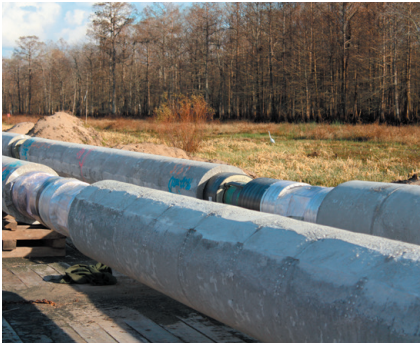
Optimized thermal insulation coated with 2.5" concrete to overcome buoyancy
