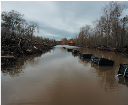
Pipeline is submerged 2 m (6 ft) below the swamp, crossing environmentally sensitive wetlands
