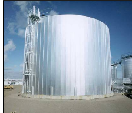
Figure 5: Typical storage tank with vertical lock-seam insulation
