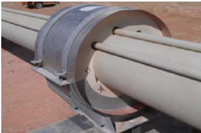
Figure 7. Engineered Thermally Isolated Pipe Anchor
