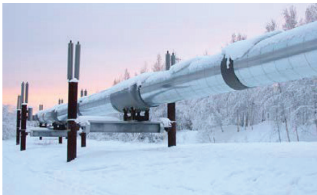
Figure 1. Alaskan Cross-Country Pipeline
