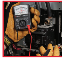
Test circuit breakers
