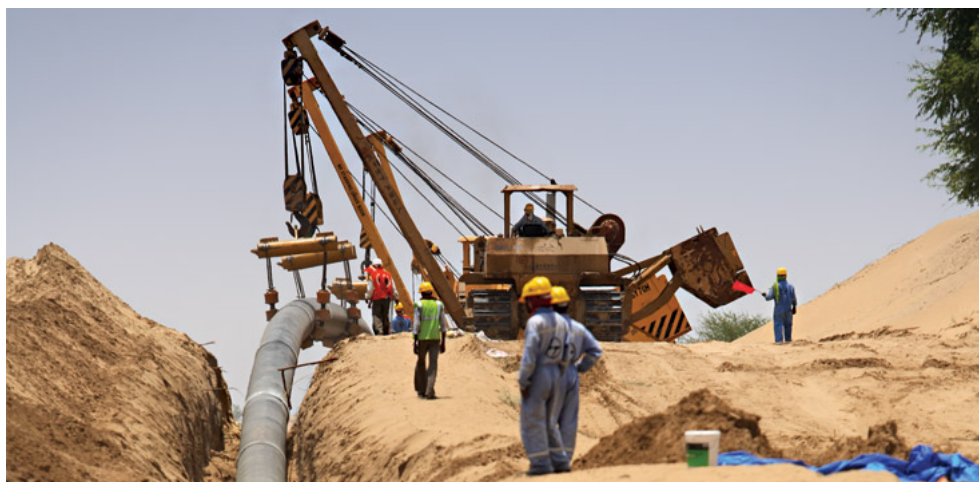
Figure 5. Construction Team Laying Pre-Insulated Pipe for Oil & Gas Development
