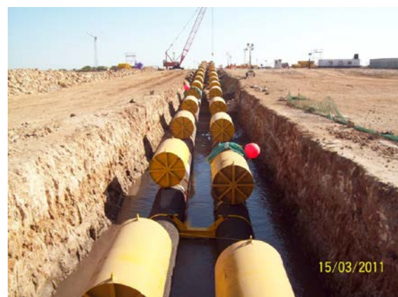
Figure 7. Pre-insulated Pipe Spool System with Flotation for Subsea Deployment
