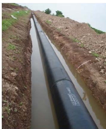
Figure 6. Pre-insulated Pipe Spool System Laid in a Flooded Trench
