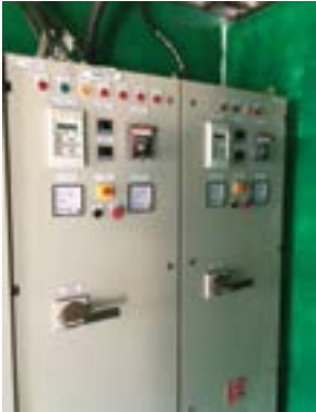
STS Control and Monitoring Panel
